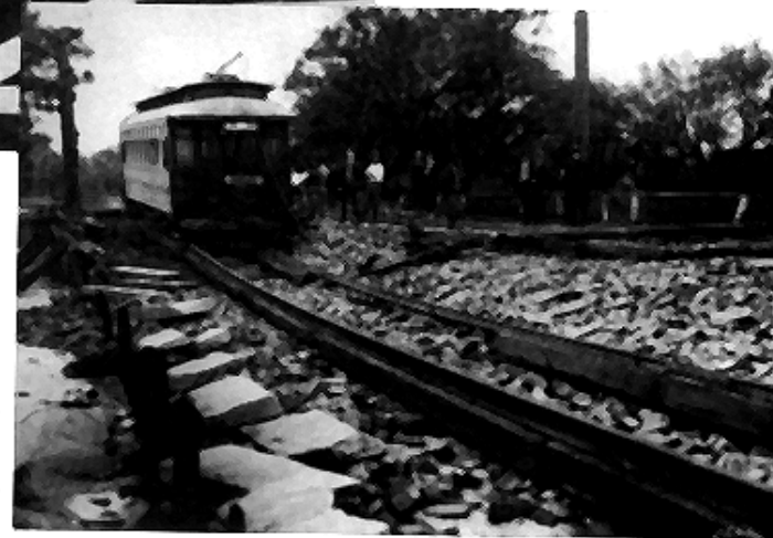
Damage on Bayshore after October 25, 1921 hurricane - Photo courtesy of Tampa Hillsborough County Public Library System
